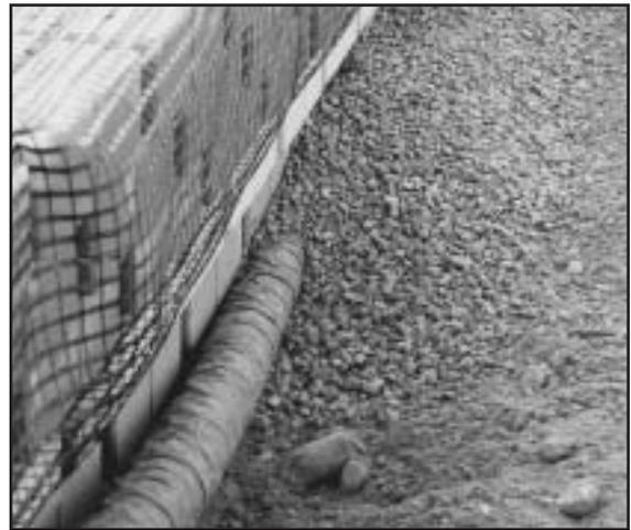
Do not place drainage aggregate behind units that will be embedded. For walls higher than three feet, a perforated drain pipe should be used to collect water along the base of the drainage aggregate. For some projects, such as shoreline applications, geosynthetic fabric may be required behind the drainage aggregate to prevent soils or sands from migrating into the drainage aggregate and wall face joints.
