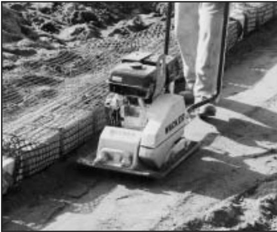
Place soil backfill beginning directly behind drainage fill in layers no thicker than six inches. Compact soil backfill, making sure that the backfill is neither too wet nor too dry. The amount and type of effort needed for adequate backfill compaction varies with soil type and moisture content. Generally, hand-operated vibratory plate compactors can be used to achieve adequate compaction of granular soils.
